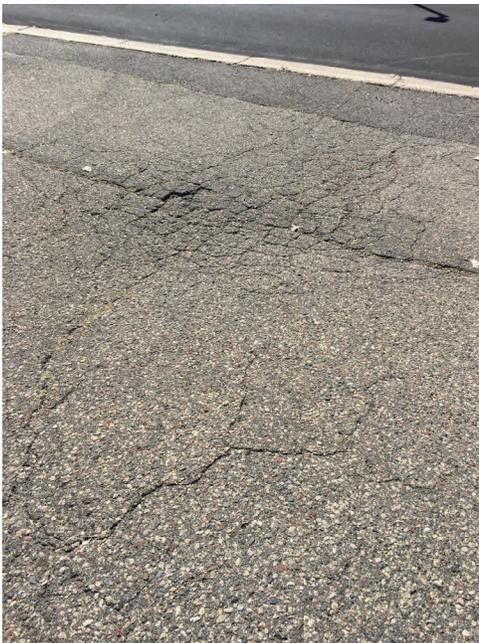
The driveway and parking lot around the headquarters building need to be replaced. The asphalt is cracked and has begun to sink in some areas. This makes the issue of snow removal increasingly challenging.
